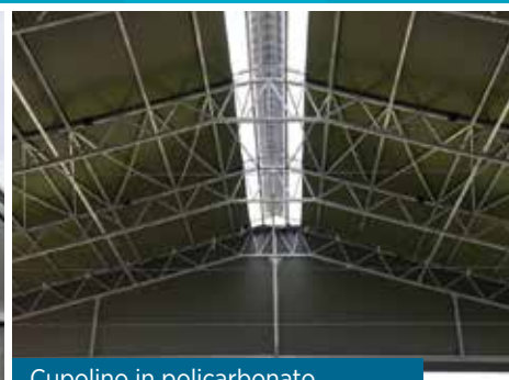
Cupolino in polycarbonato Polycarbonate ridge opening
