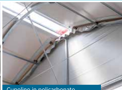
Cupolino in polycarbonato Polycarbonate ridge opening
