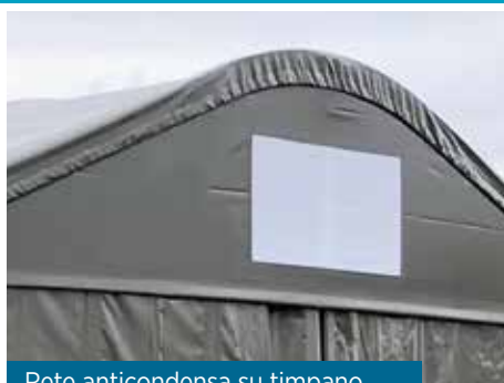
Rete anticondensa su timpano Anti-condensation net on the gable
