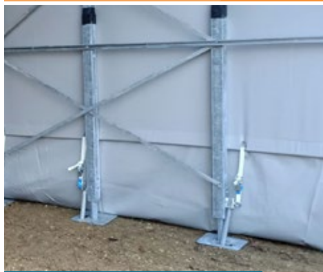
Anchorage au sol Ground fastening
